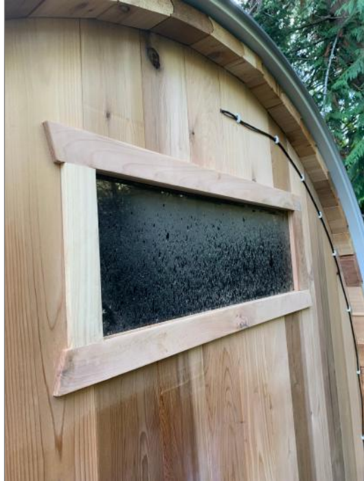
Figure 1 - Approximate hole placement for Temp Sensor.
